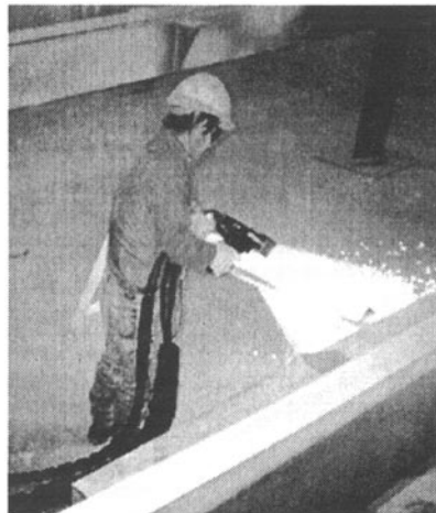
Fig. 4 Aluminum arc spraying in a Canadian fabrication shop.
